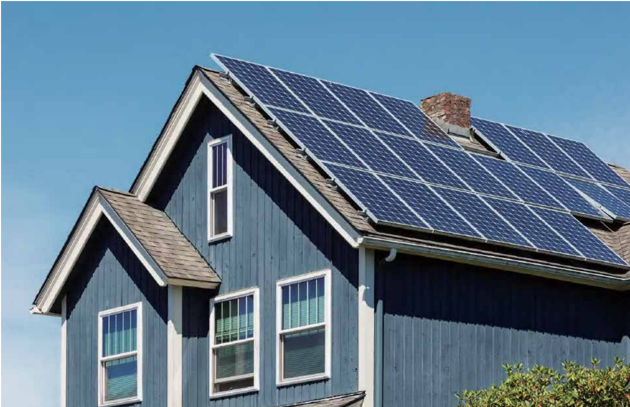
Rooftop Power Generation
